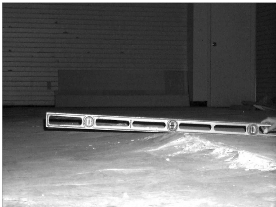
Figure 31 –Vertical displacement of floor from pyrite oxidation, from (Carter 2002b).
