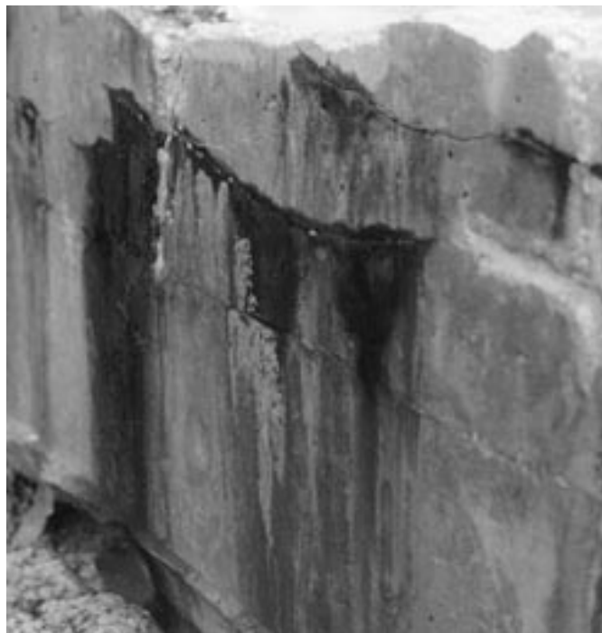
Figure 29 – Concrete degradation resulting from “sulfate attack” and corrosion. Photo from corrosion.ksc.nasa.gov/ .
