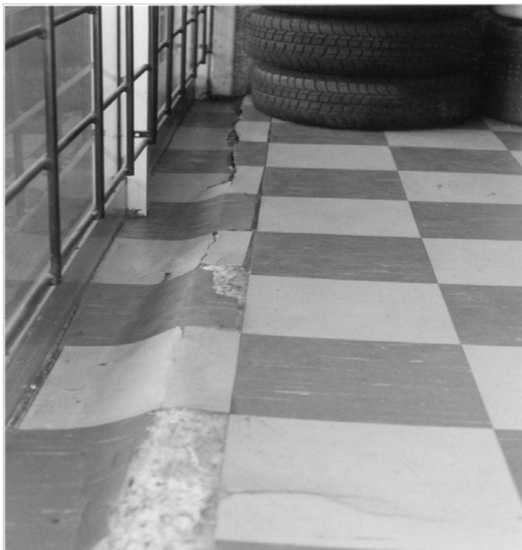
Figure 30 – Floor heave resulting from pyrite oxidation, from (Carter 2002b).
