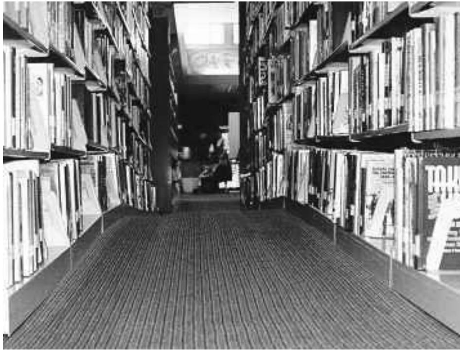
Figure 14 – Sulfide-induced heave of library floor and bookshelves at Johnson City Public Library, Johnson City, Tennessee.
