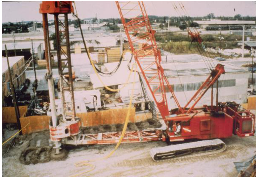
Equipment Installing a Block-Type Deep Mixing Pattern (Figure from Elias et al. (2006))
