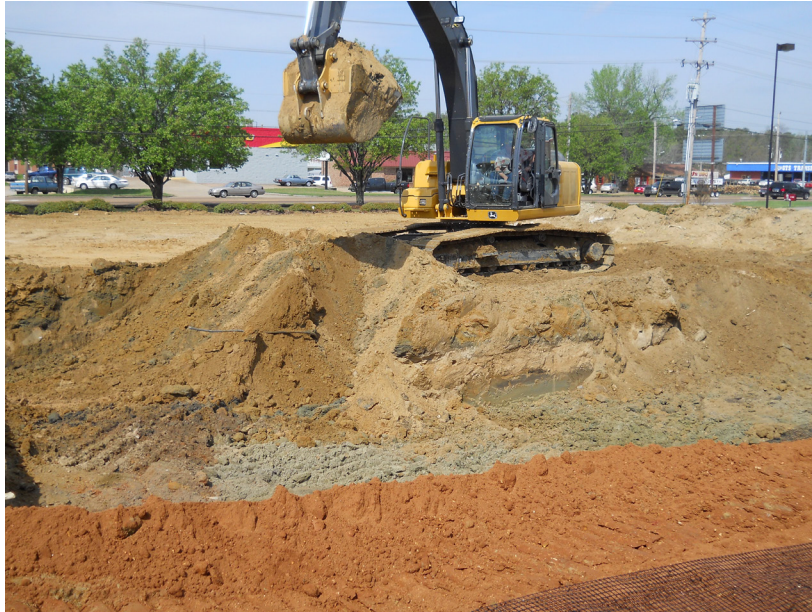
Excavation of Unsuitable Soil using Hydraulic Excavator in Columbus, Mississippi (Photograph courtesy of David M. Coleman)
