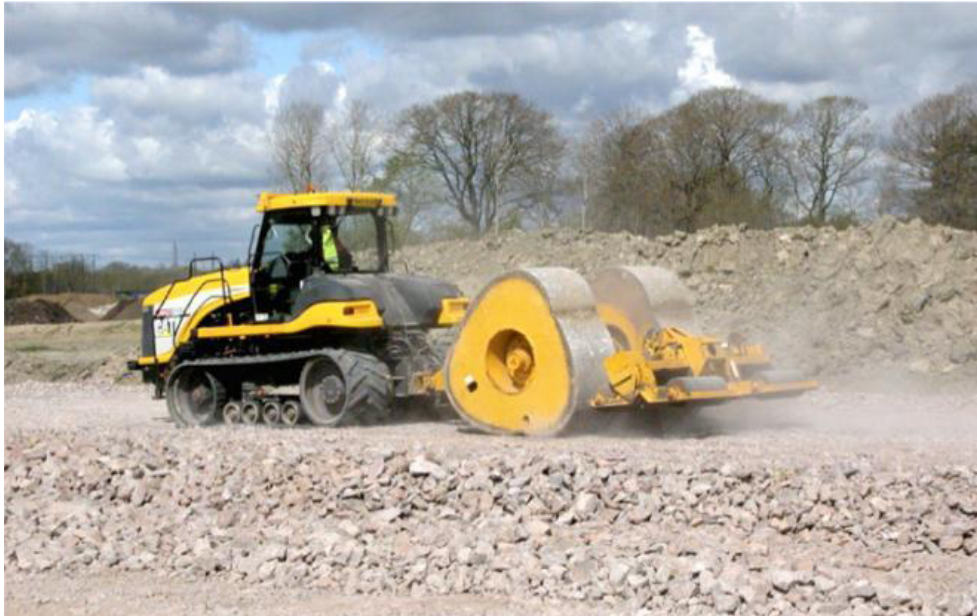
Landpac 25-kJ Three-Sided Impact Roller (Photograph courtesy of Landpac® (www.ladnpac.co.uk))
