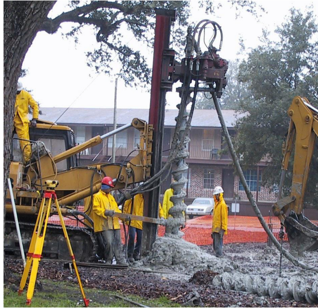
Low Headroom CFA Pile Application
