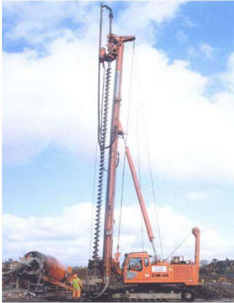
CFA pile rig
