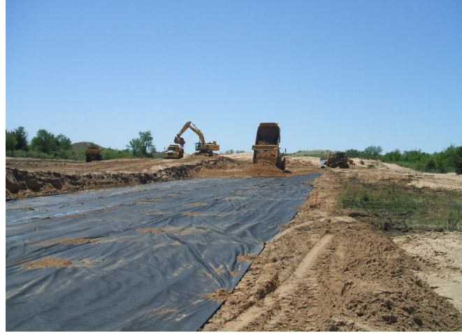
Placement of geosynthetic in roadway (Courtesy of Kansas Department of Transportation)
